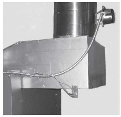
Figure E: Blocked Vent Switch Installation
