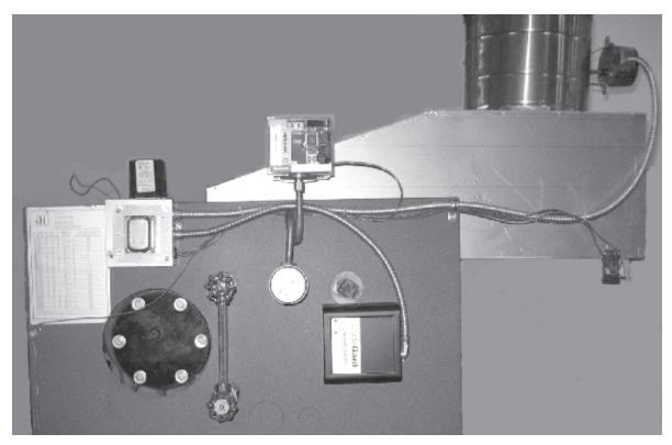
**Figure D: Steam Boiler Control Installation**
